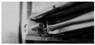
8. Minimum Gas Pressure Adjustment. Attach manometer to burner test point (see picture above) Set water flow selector fully clockwise (hot position). Move gas slide to left side, single flame symbol, open hot tap fully. Turn adjustment screw (Position C in picture below) located on left hand side of gas valve at a 45° angle to correct pressure. Anti clockwise to decrease minimum burner pressure.
